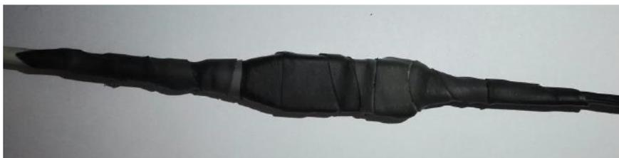
g. Now use the insulation tape to cover the rubber tape
